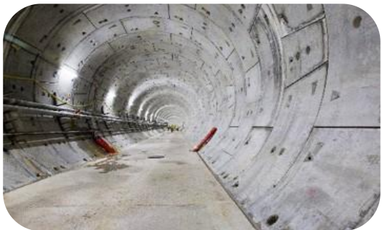
MRT Tunnel Lining with 20% Fly Ash
