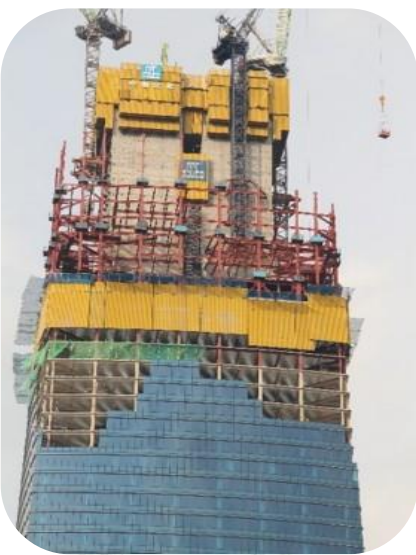
The Exchange 106 using High Strength Grade 75 concrete with 50% OPC + 30% GGBS + 20% PFA
