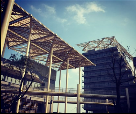
SDTI E-Waste Recycling Infrastructure with Façade and canopy system made from old computers
