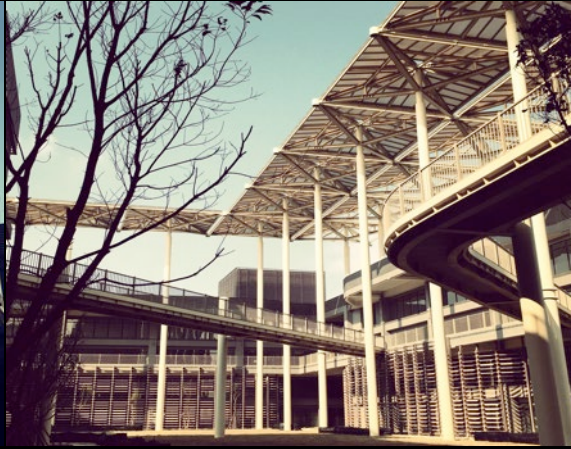
SDTI E-Waste Recycling Infrastructure with Façade and canopy system made from old computers
