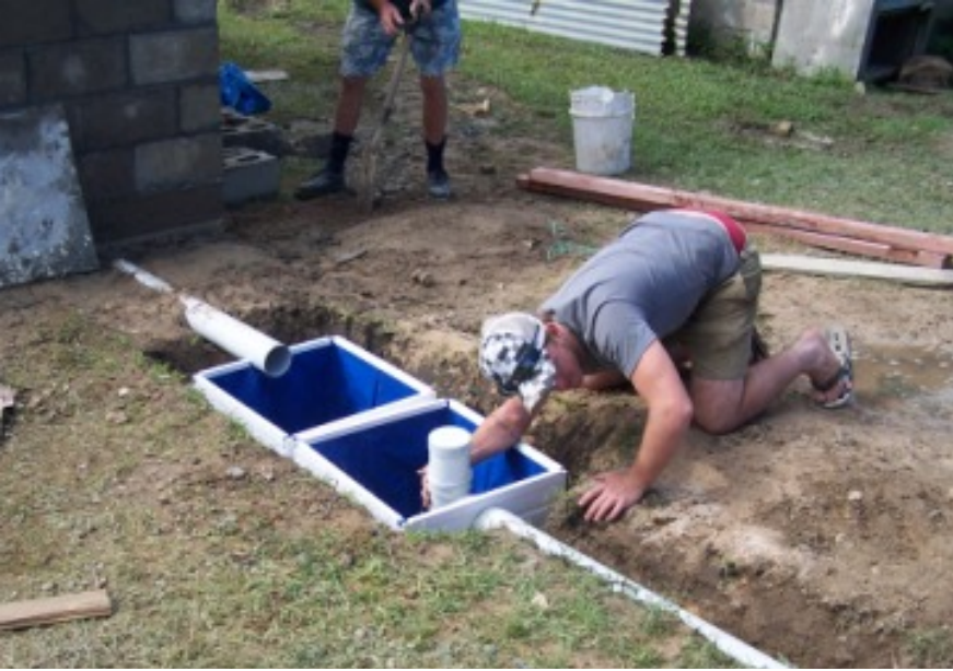
BIPU septic chambers for developing countries
